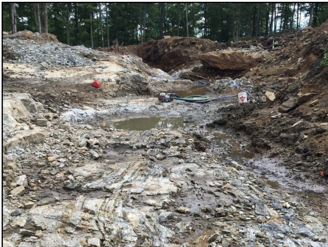
Figure 9-8: Example of a Trenched Area with Banded Mineralization at VN6
